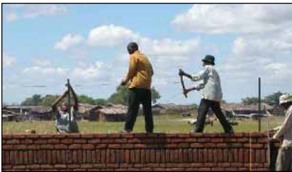
LM crew stretching wire for the fence
